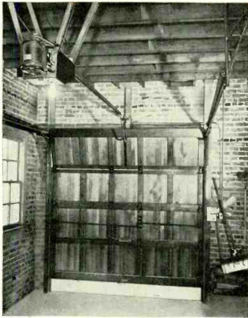
Left, completed installation of operator in garage.
